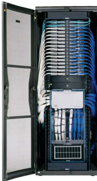
(Nexus 7010 "Heavy Copper" Pre-Configured Physical Infrastructure shown)
