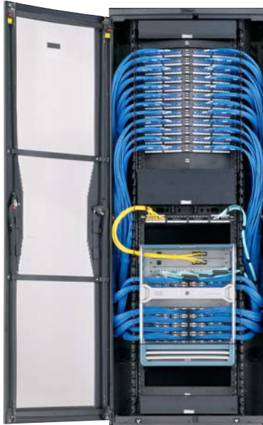
(Nexus 7009 "Heavy Copper" Pre-Configured Physical Infrastructure shown)
