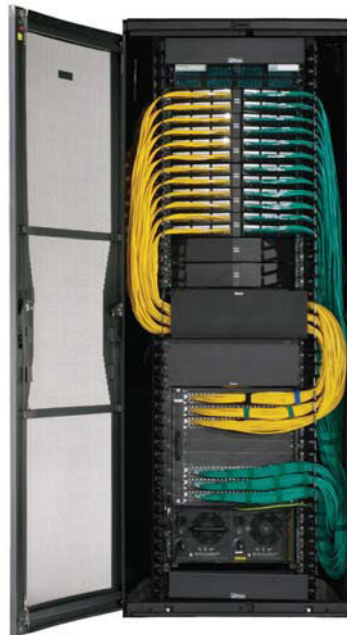
(Catalyst 6509 "Heavy Copper" Pre-Configured Physical Infrastructure shown)
